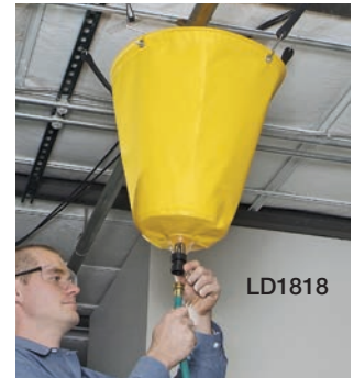
Installation is easy – simply hang from overhead pipes.
