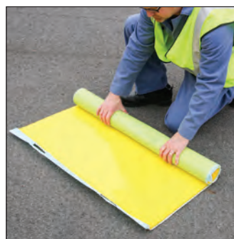
Once clean, roll the cover poly side up onto its silicone fabric.
